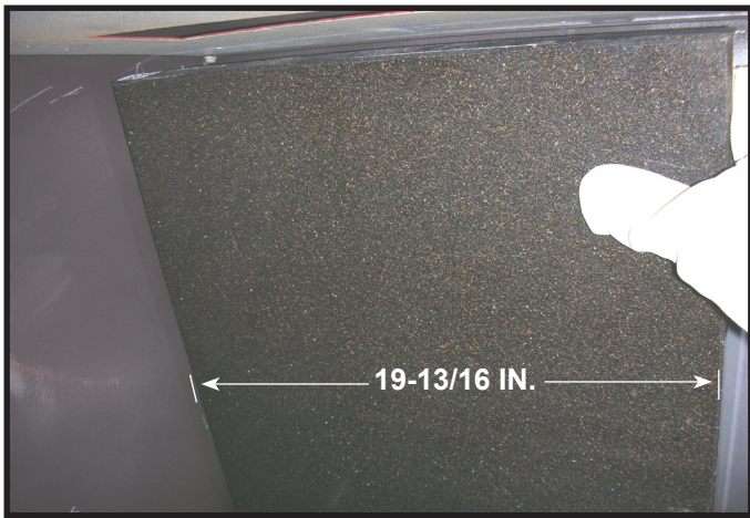
Figure 11. Installing First Back Panel Granite Piece.
